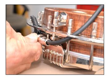
10. Cable-tie the jack onto 2 tuning lugs and tighten the cable ties with needle-nose-pliers.
